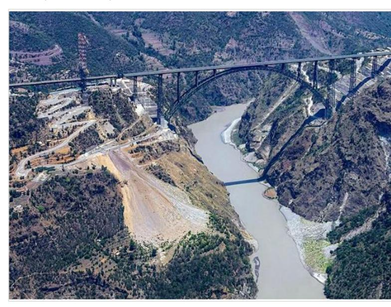
• Built at a cost of around Rs 1,400 crore, the Chenab bridge is the **highest rail and arch bridge in the world** with a dock height of 359 meters from the river bed, 35 meters taller than Paris's iconic Eiffel Tower.
